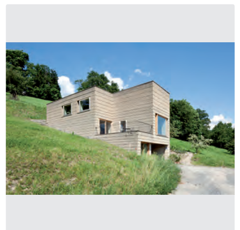
Roger Boltshauser and Martin Rauch Haus Rauch | Rauch House | Schllins Photo: Beat Bühler
